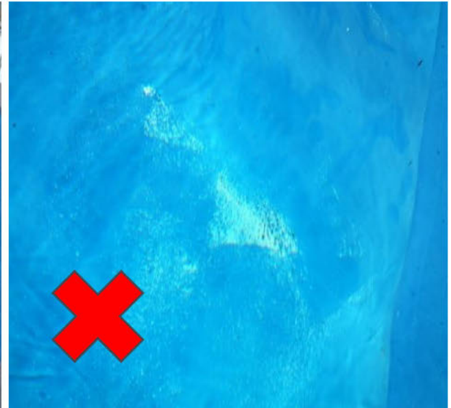
Figure 2. Not enough uniform spreading out and laying off, worn away too soon in some areas. Pool owner will say the paint is not good. Then what? Compare with pic on 1 st page.
