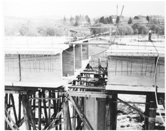
Figure 2.16 Multi-webbed box segments from adjoining spans placed over pier before preliminary tensioning. (Source: National Library of Australia, nla.obj-145675579-1)
