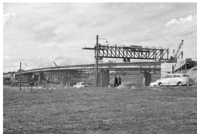
Figure 2.18 Bridge superstructure self-supporting after post tensioning. The timber falsework is in process of being removed. (Source: National Library of Australia, nla.obj-143758408-1)
