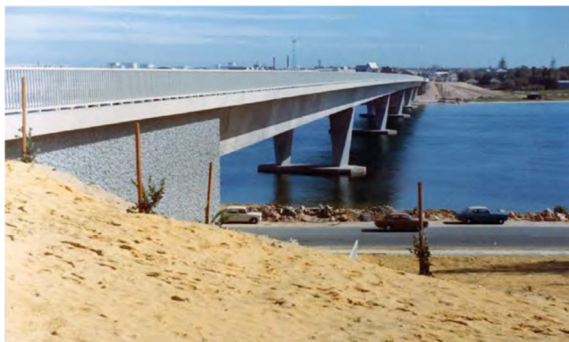
Figure 13 Stirling Bridge over the Swan River. The segment depth and span length decrease progressively. (Source: J. O. Clough & Son, Engineers Australia)
