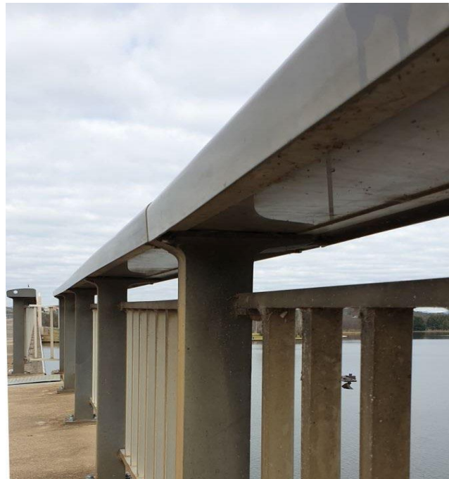
Figure 3.7 Detail of integral handrail lighting of the Commonwealth Avenue Bridge. (Source: K Baker, 2020)
