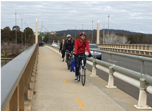
Figure 2.23 Addition of cyclist safety rails above the roadway rails on the eastern side of the bridge. (Source: K Baker, 2020)
