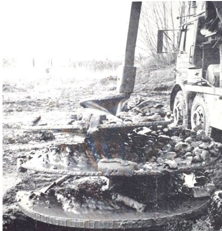
Figure 2.10 Boring the bridge pile, which was 2 metres in diameter. (Source: Hornibrook, 1964)
