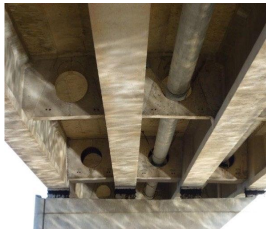
Figure 3 Under side of Kings Avenue Bridge demonstrating an industrial appearance with four 'T' beams and exposed pipes passing through diaphragms. (Source: K Baker, 2013)
