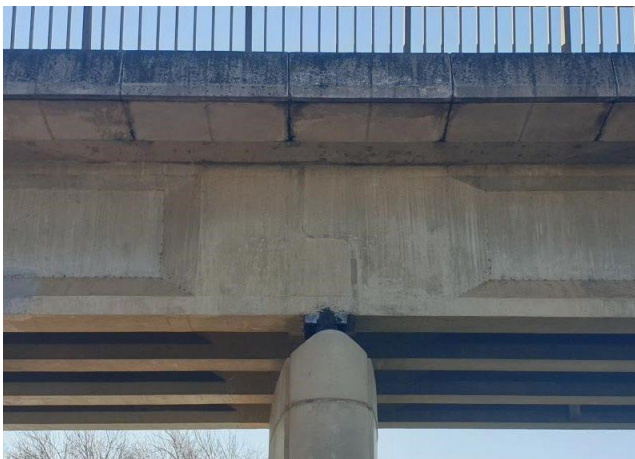
Figure 2 Half lapped join of precast beams over bearing on pier. (Source: K Baker, 2020)
