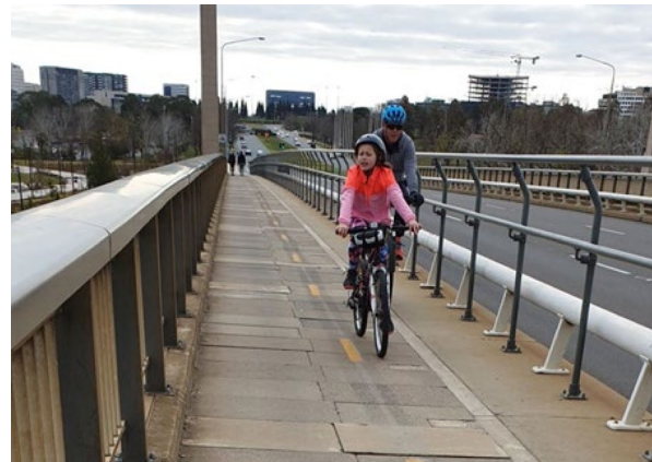
Figure 2.24 Addition of temporary cyclist safety rails alongside the roadway rails on the western side of the bridge. (Source: K Baker, 2020)
