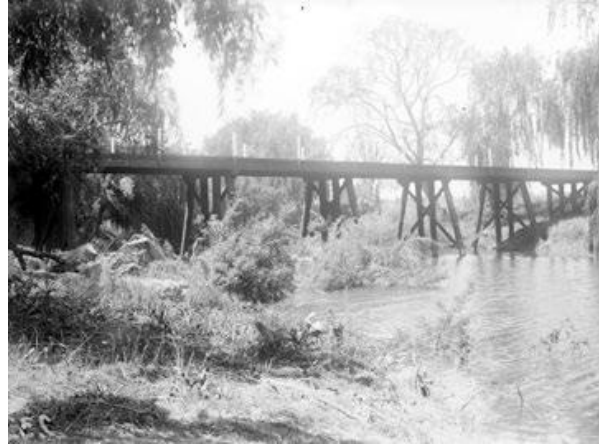
Figure 2.2 First Commonwealth Avenue Bridge, which was destroyed in the 1922 flood. (Source: National Australian Archives, A3560, 232).
