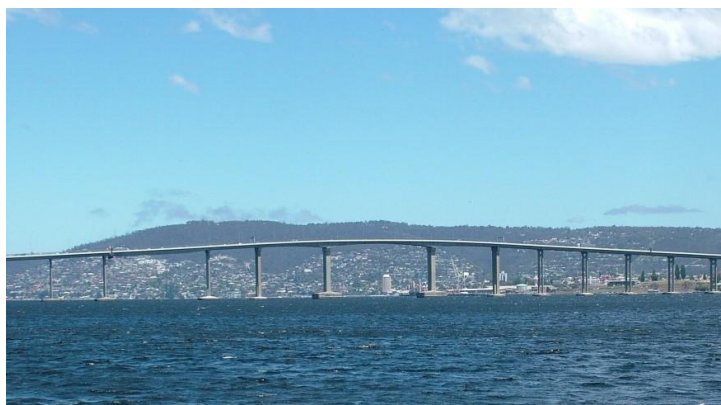
Figure 11 The Tasman Bridge over the Derwent River was built at high level to accommodate shipping lanes, with multiple spans across the river and approaches. Consisting of a superstructure of simply supported prestressed concrete beams. Some spans were replaced with steel after major damage by a ship. (Source: Creative Commons Phil Wardle)
