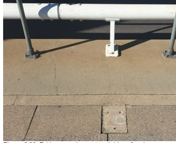
Figure 2.22 Evidence on the western bridge of cycleway widening and relocation of the safety rails. (Source: K Baker, 2020)
