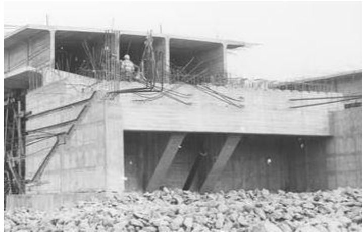
Figure 2.11 Bridge abutment, supporting an end span of the superstructure. (Source: National Library of Australia, c1962–1963, nla.pic-an24577607-v)
