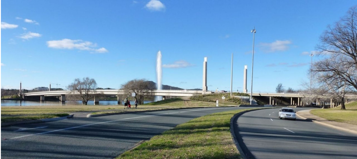
Figure 4 Graceful low arch of Commonwealth Avenue Bridge viewed from Flynn Drive. (Source: K Baker, 2013)
