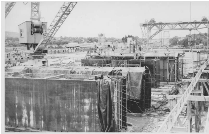
Figure 2.15 Cast multi-webbed box segments curing before placement on timber falsework. Note the projecting reinforcement for addition of cantilever walkway once in place. (Source: National Library of Australia, nla.obj-145675273-1)
