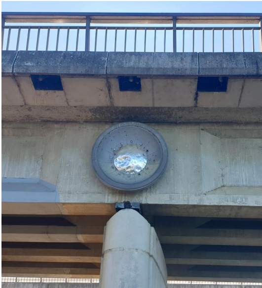
Figure 3.4 Kings Avenue Bridge lighting in handrail and below to light roundel. (Source: K Baker, 2020)
