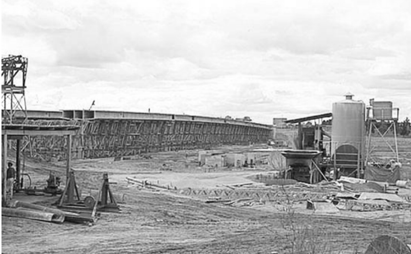
Figure 2.13 Multi-webbed box segments in place on top of the timber falsework. The concrete batching plant and casting yard are in the foreground. (Source: National Library of Australia, nla.obj-143758146-1)
