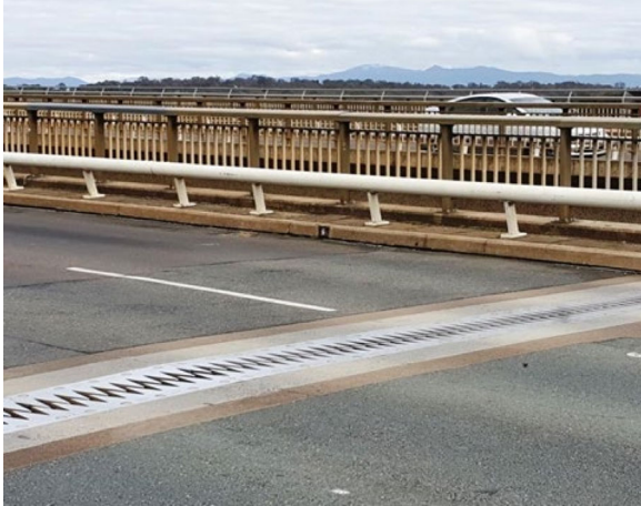
Figure 2.21 Safety rails mounted on the concrete kerbs at the edge of the roadways. (Source: K Baker, 2020)
