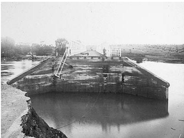
Figure 2.5 Commonwealth Avenue Bridge, showing flood damage in 1925. (Source National Australian Archives, 3560,7668)
