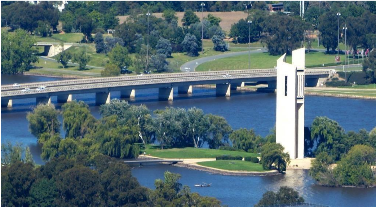
Figure 1 Kings Avenue Bridge from Mount Ainslie with Carillon and Aspen Island in the foreground. It has shorter spans and broader piers than Commonwealth Avenue Bridge. (Source: K Baker, 2013)
