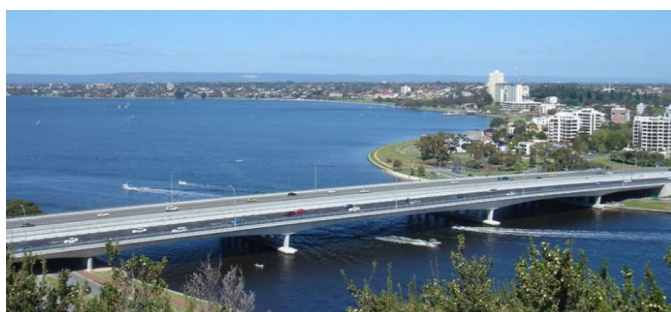
Figure 7 The Narrows Bridge over the Swan River, Perth WA. A later duplicate road bridge is in the foreground. (Source: Wikipedia Creative Commons Mailer Diablo)
