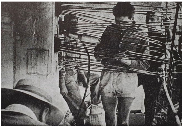
Figure 7 Transverse Stressing. Pier Segment Diaphragm.
