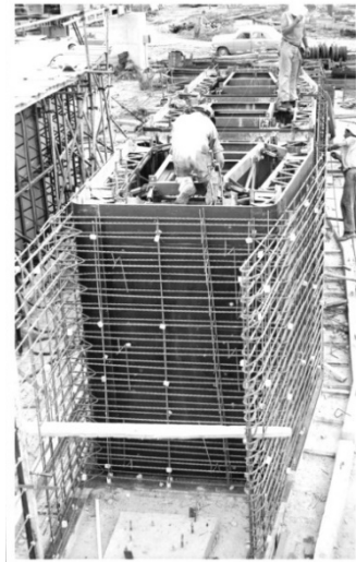
Figure 2.14 Reinforcement placed around inner form of box segment. (Source: National Library of Australia, nla.obj 24577602)
