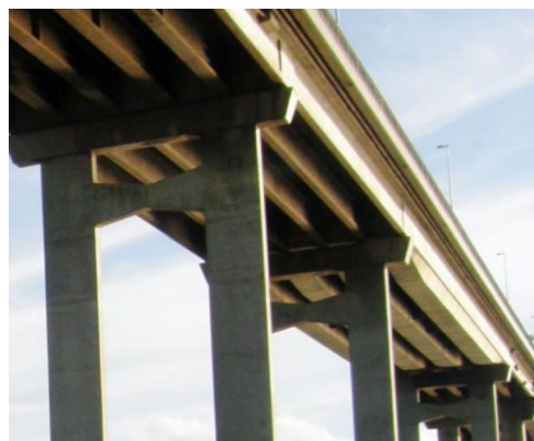
Figure 12 Underside of Tasman Bridge showing the six parallel concrete 'I' beam structure with steel replacement in the adjacent span. (Source: Creative Commons Wiki Ian)
