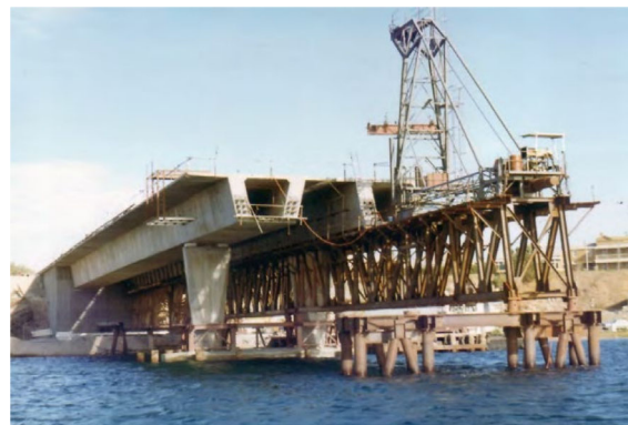
Figure 14 Side-by-side 'T' segment box girders structure during construction. (Source: J. O. Clough & Son, Engineers Australia)
