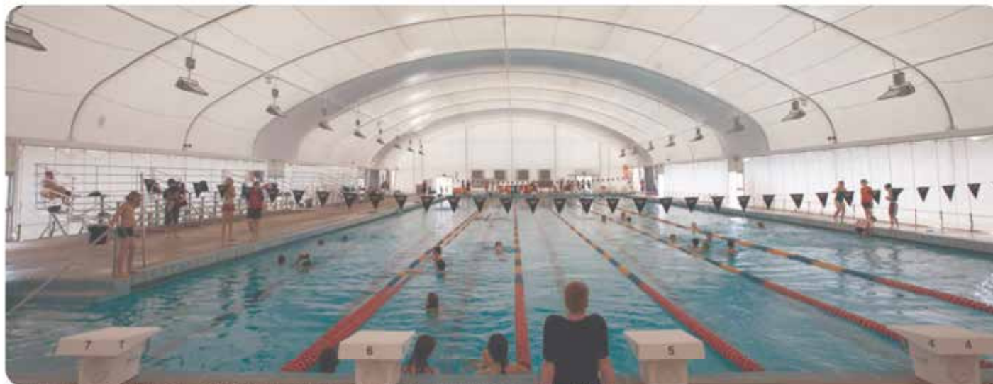
Figure 1: Photograph: Canberra Olympic Pool 50m lap pool under pneumatic structure, 2018, Canberra Olympic Pool, https://www.canberraolympicpool.com.au/getmedia/2d0eaf70-6197-4202-898a-bfcc9e62d668/COP-1.png?ext=.png
