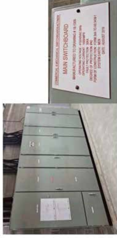
Figure 32 Main Switchboard
