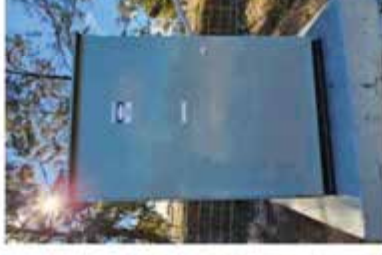
Figure 31 Evo Energy 500KVA padmount substation and LV pillar
