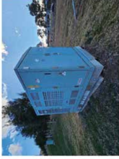
Figure 31 Evo Energy 500KVA padmount substation and LV pillar
