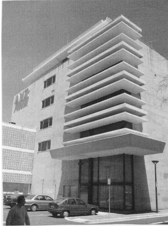
Figure 6. Smaller series of shades on northern façade – viewed from Hobart Place.
