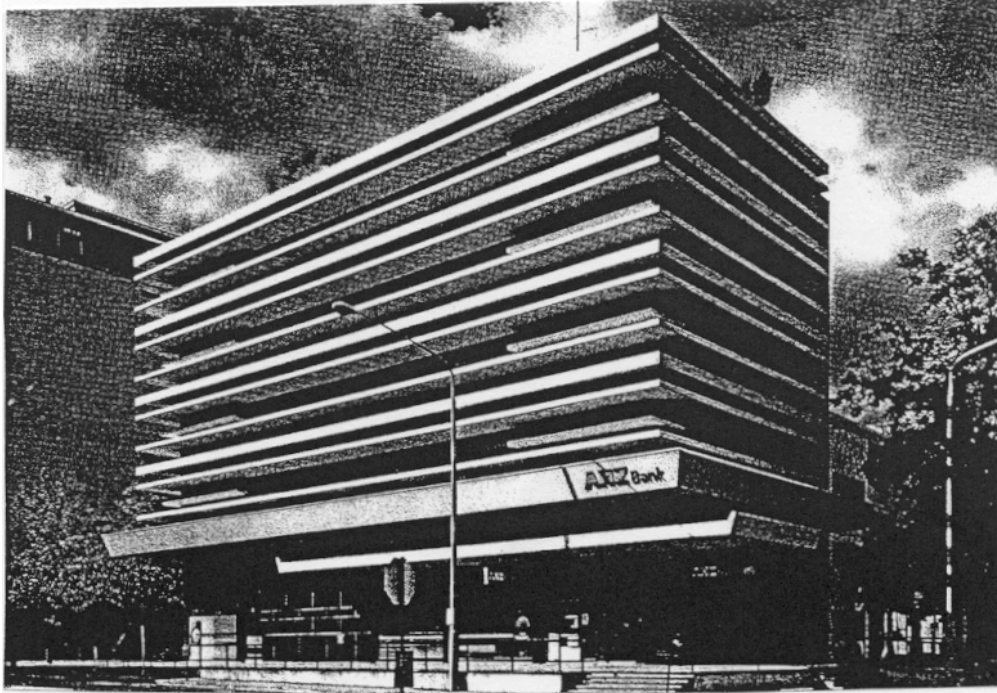
Figure 8. The former ES & A Bank Building, Malvern, Victoria, designed by Stuart McIntosh (photo: Heritage Victoria website)
