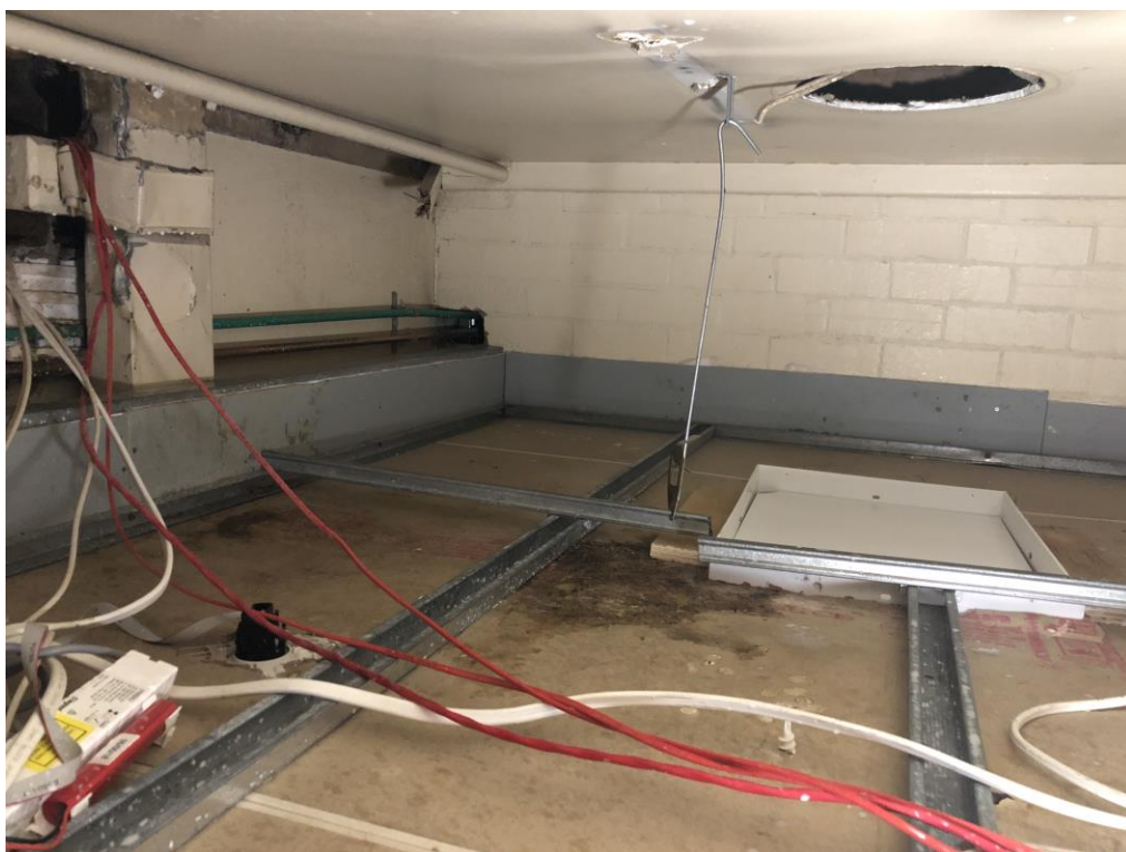
Photograph 1: Storeroom ceiling void following lead dust removal.
