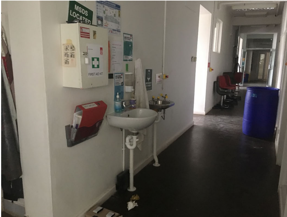
Photograph 3: Sample water location W04, Hallway.
