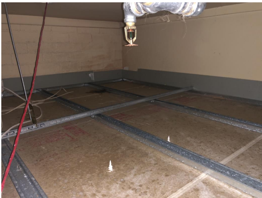
Photograph 2: Storeroom ceiling void following lead dust removal.
