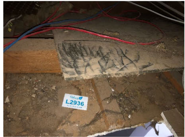
Figure 2: Surface sample L2936 location in corridor ceiling space adjacent "Aquatint" room
