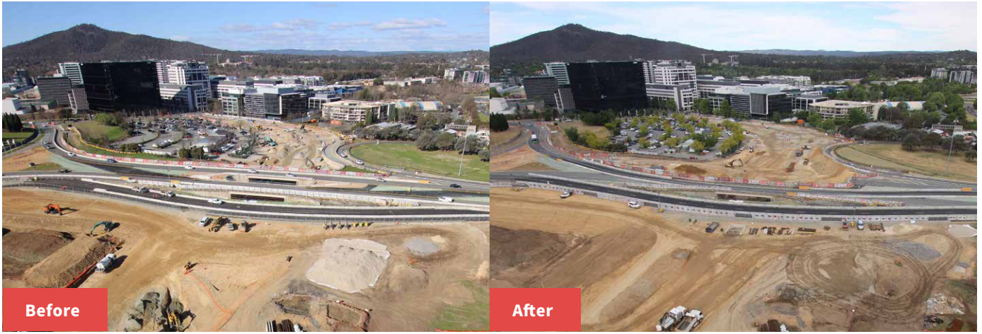
Side track before and after.
