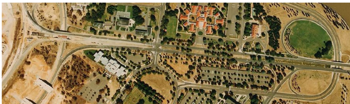
Figure 3.14 The southern end of Commonwealth Avenue with Parliament House under construction, 1985. (Source: ACTmap)
