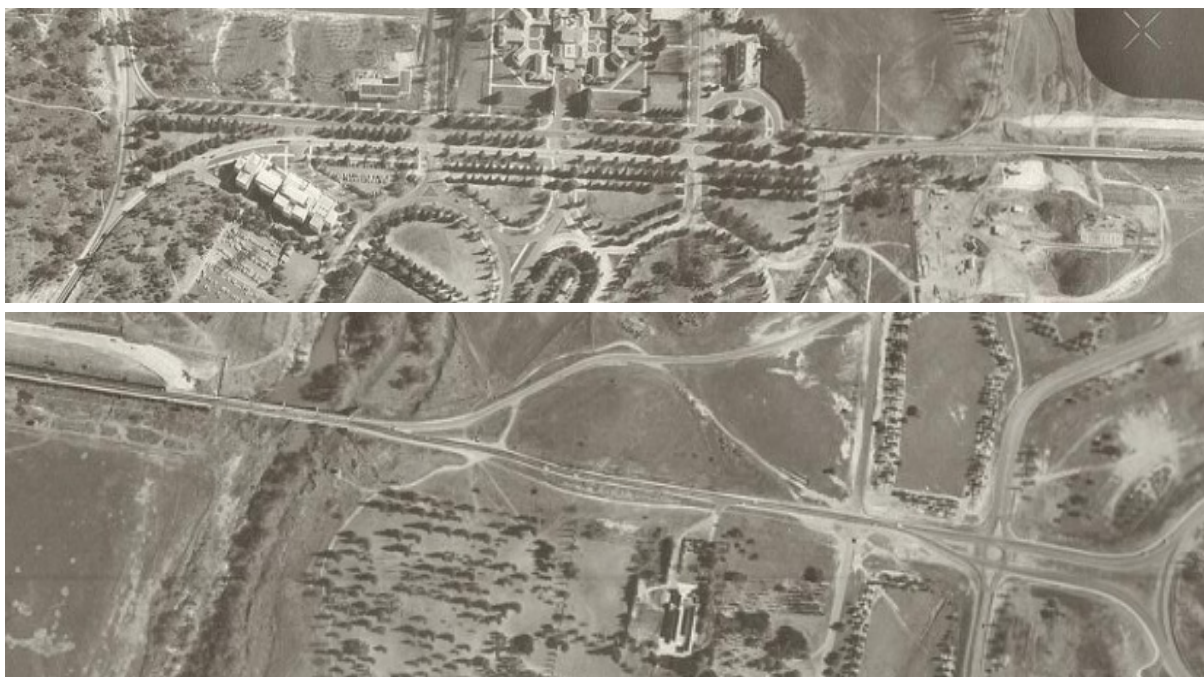
Figure 3.11 Detail of a 1961 aerial of Commonwealth Avenue, showing southern (top) and northern (bottom) sections of the avenue. (Source: ACTmapi).
