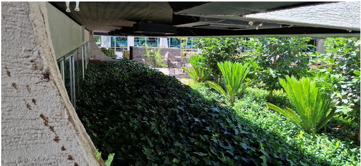
Figure 8 The only remaining original Taglietti designed light fixtures in 2026 are located under the eaves between the café and courtyard, facing west.
