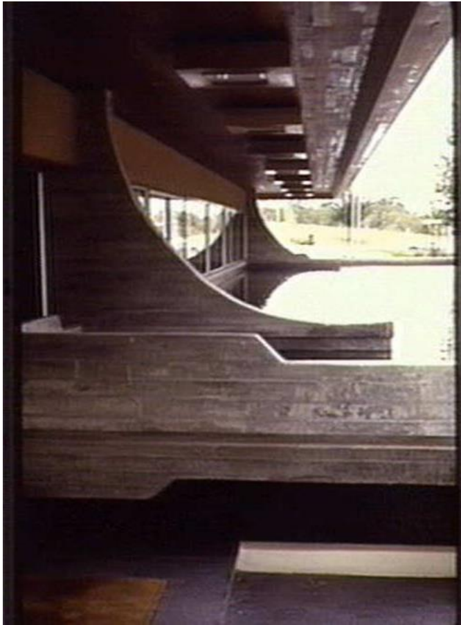
Figure 7 The northern end of the original pond under the eaves of the lobby (Wille, P., & Taglietti, E. (1966). Associated Chamber of Manufacturers Conference Centre. Brisbane Avenue. Barton. Canberra. A.C.T. Dr. Enrico Taglietti. 1966.)
