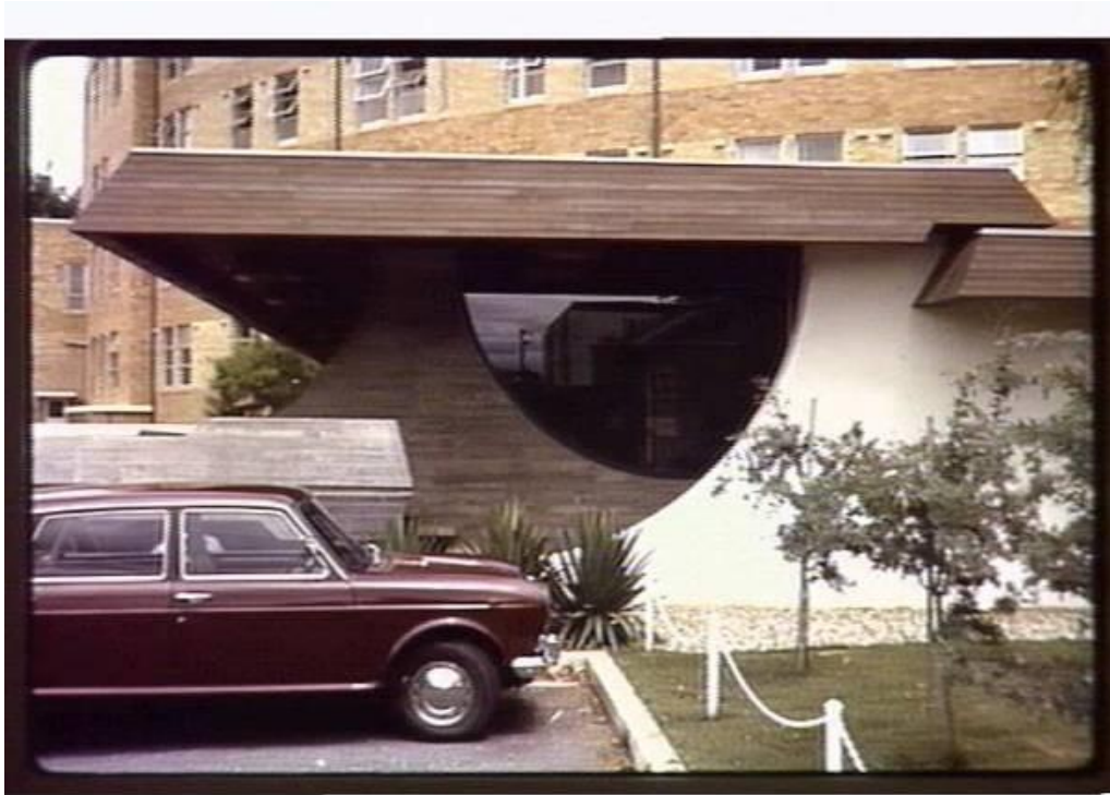
Figure 5 Original east end concrete features and wood fascias (Wille, P., & Taglietti, E. (1966). Associated Chamber of Manufacturers Conference Centre. Brisbane Avenue. Barton. Canberra. A.C.T. Dr. Enrico Taglietti. 1966.)
