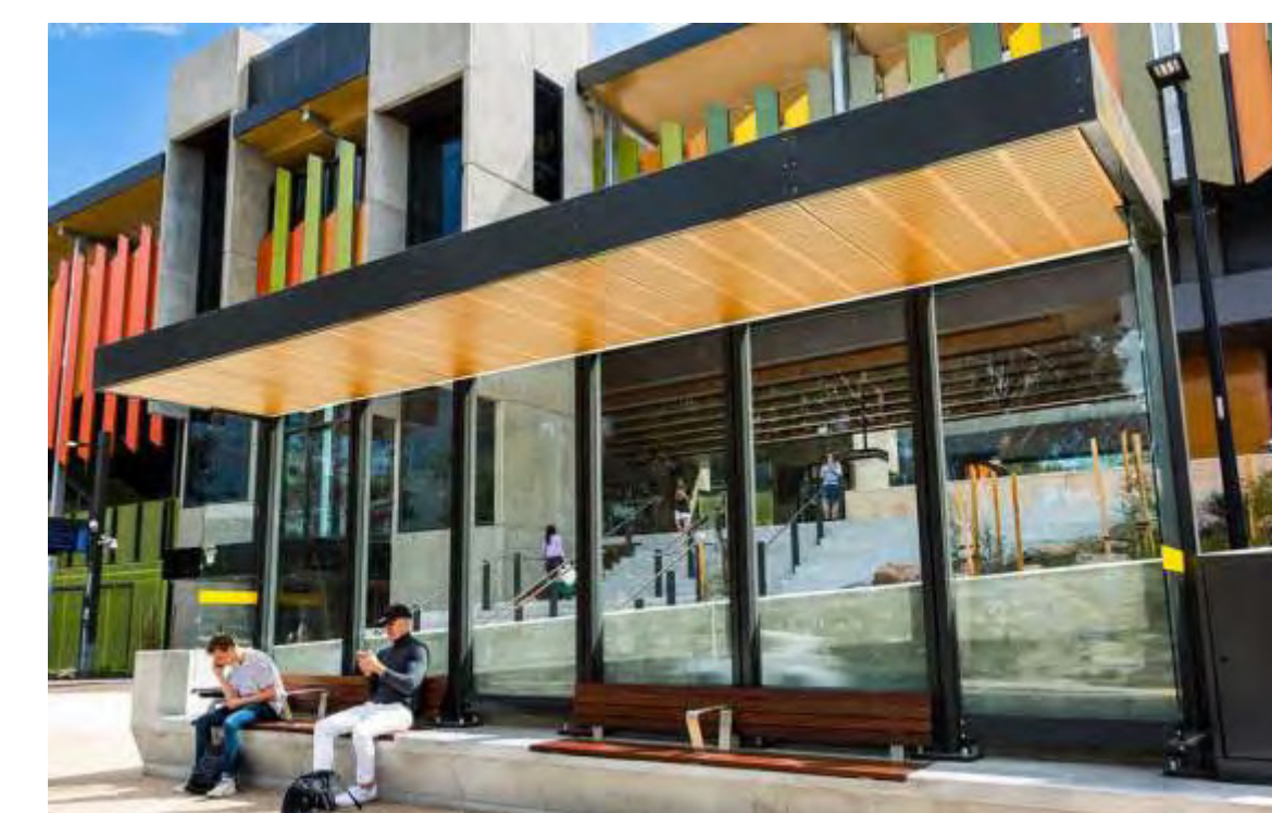
Rosanna Station - Jacobs 2018 Image Source - https://www.stoddart.com.au/infrastructure_references
