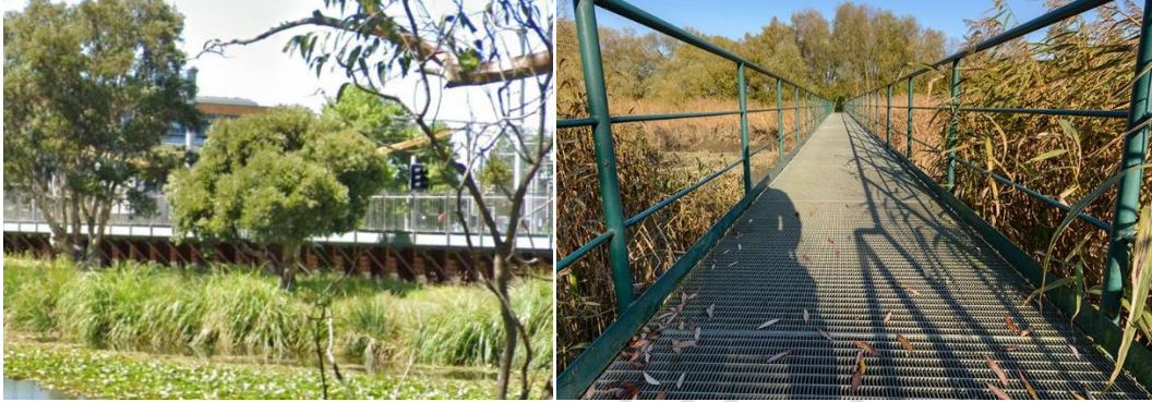
Figure 14 - Shared path on structure over swale at Alison Road (Sydney) Figure 15 - Example of walkway
