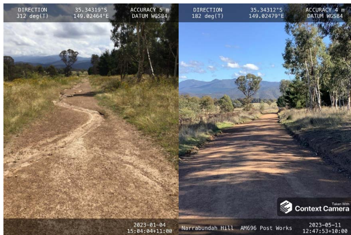
Figure 29: AM696 Before / After – large ruts removed from road, drainage redirected, regraded.
