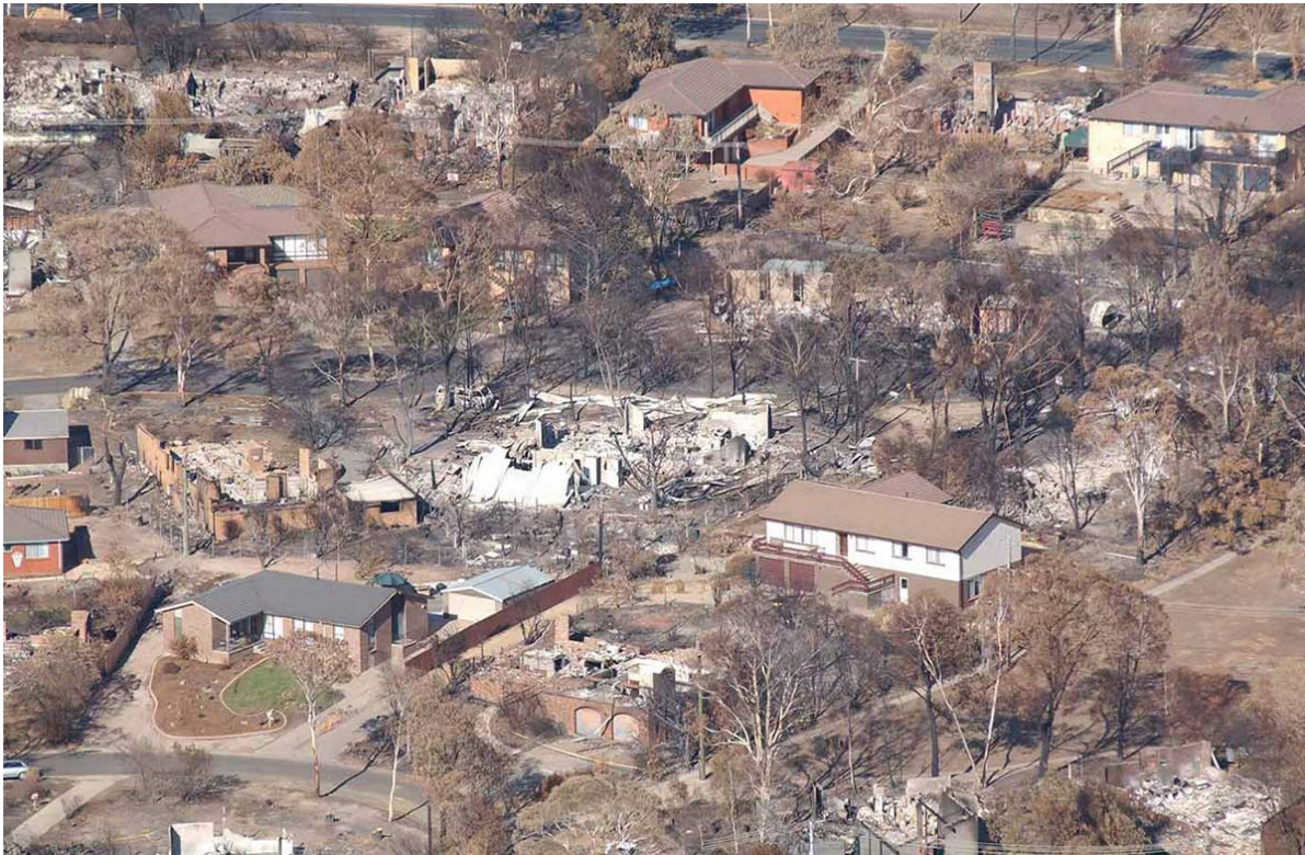
Figure 24: Homes destroyed in Duffy looking towards Eucumbene Drive (Source: National Museum Australia)
