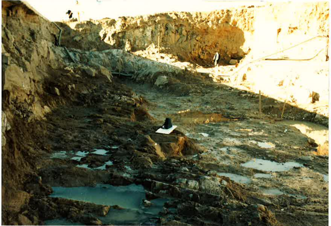
PHOTOGRAPH 6 Southern Abutment, general foundations downstream of cut-off trench. June, 1986
