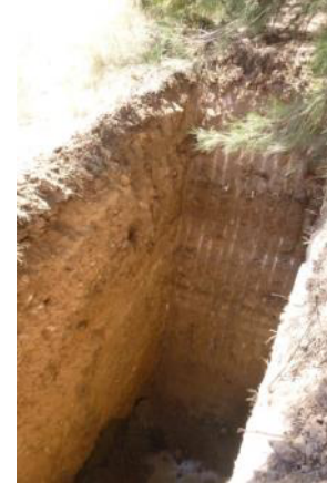
Test Pit T04 –U/S end of pit
