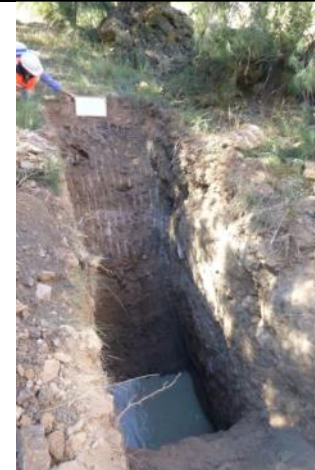
Test Pit T09 – U/S end and left side wall of pit
