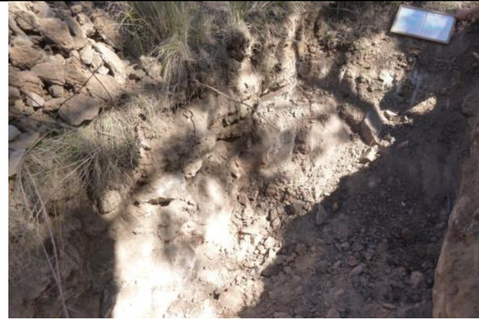
Test Pit T10 – R/H end and D/S side wall of pit (2)
