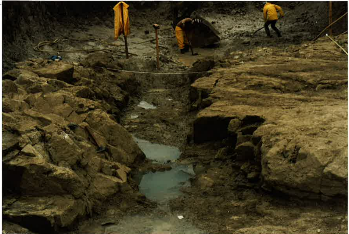
PHOTOGRAPH 2 Northern Abutment, view downstream. June, 1986
