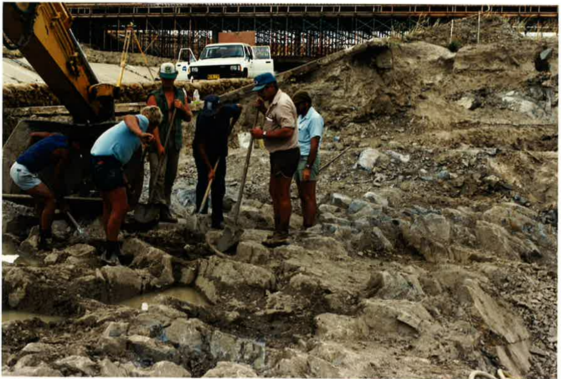
PHOTOGRAPH 7 Central Channel, east side, clean up in progress. February, 1987
