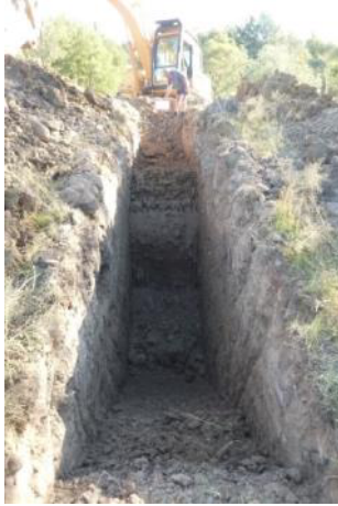
Test Pit T06 – D/S end of pit
