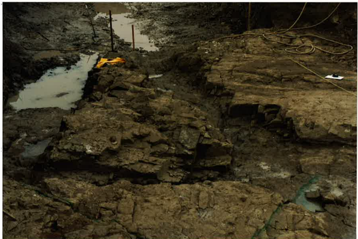
PHOTOGRAPH 3 Northern Abutment, detail of abutment foundation. June, 1986
