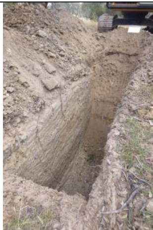
Test Pit T02 – D/S end and left side wall of pit
