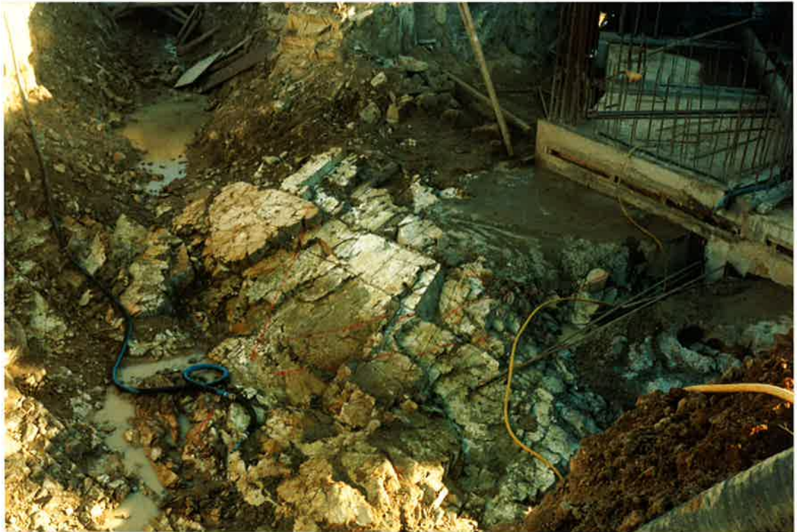
PHOTOGRAPH 12 Southern Abutment, showing large gently dipping joints, view south. May, 1987
