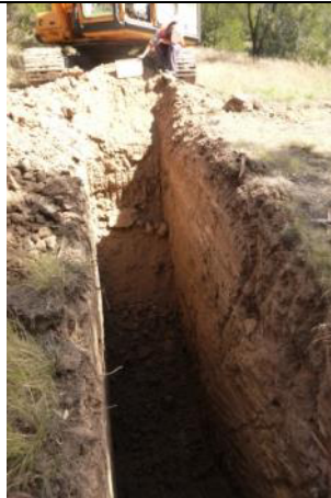
Test Pit T03 – D/S end of Pit
