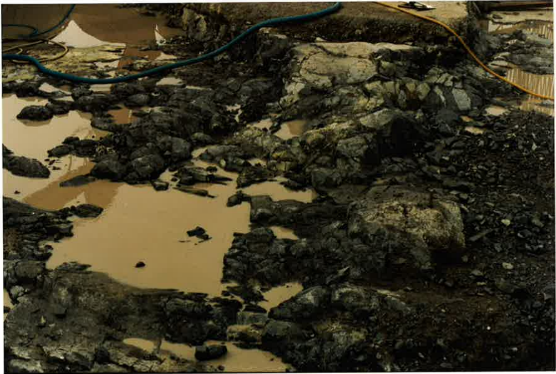
PHOTOGRAPH 10 Central Channel, labyrinth wall foundations during clean up. February, 1987
