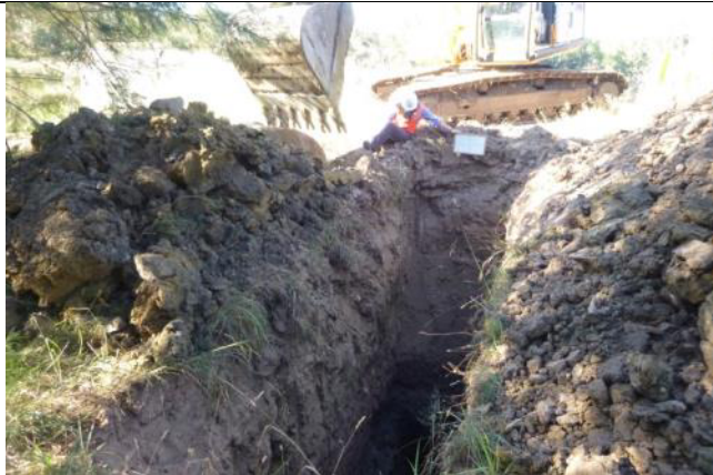
Test Pit T07 – D/S end of pit and excavated spoil
