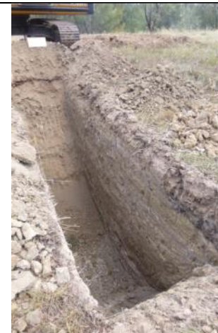
Test Pit T02 –D/S end and right side wall of pit
