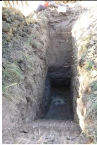
Test Pit T07 – Base of pit and D/S end of pit
