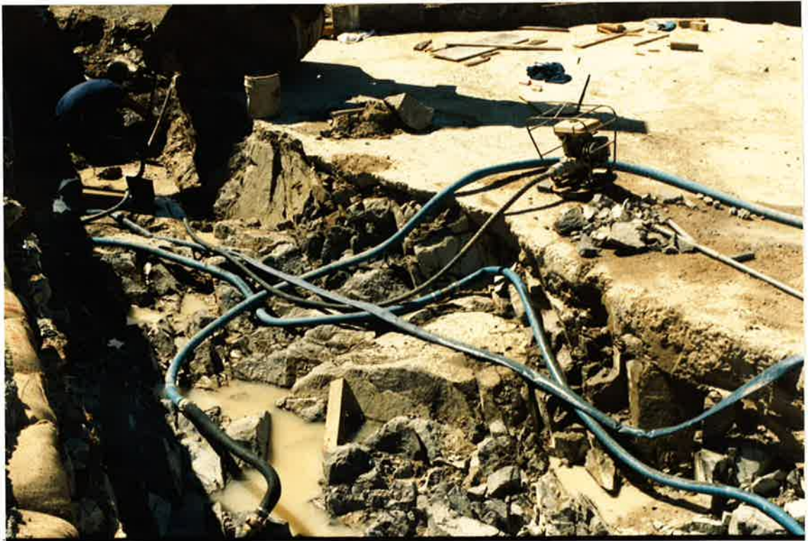
PHOTOGRAPH 9 Central Channel, east side, clean up of foundation trenches. February, 1987
