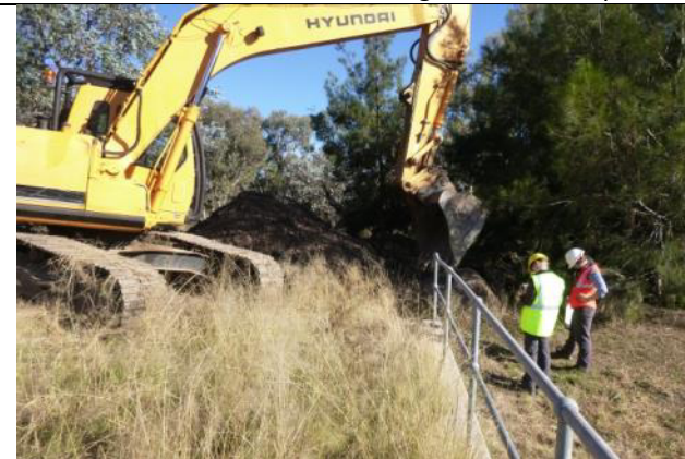
Test Pit T07 – Pit location relative at end of concrete wall
