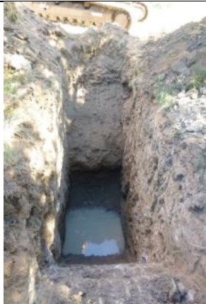
Test Pit T09 – D/S end and base of pit
