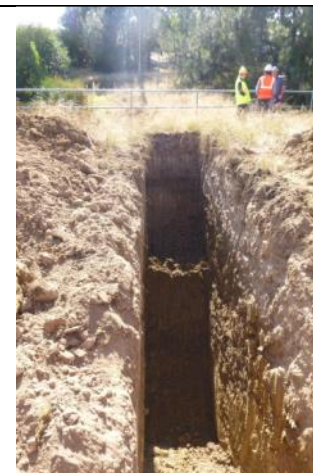
Test Pit T05 – D/S end and left side wall of pit
