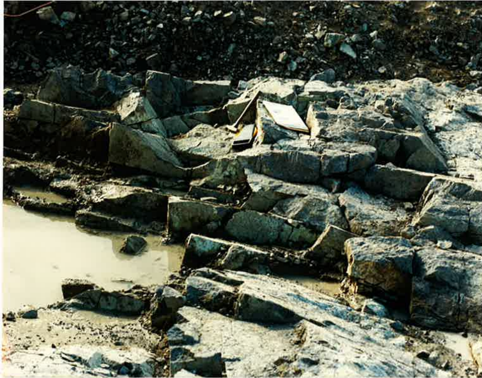
PHOTOGRAPH 14 Central Channel, west side, detail of shallow dipping joints. July, 1987
