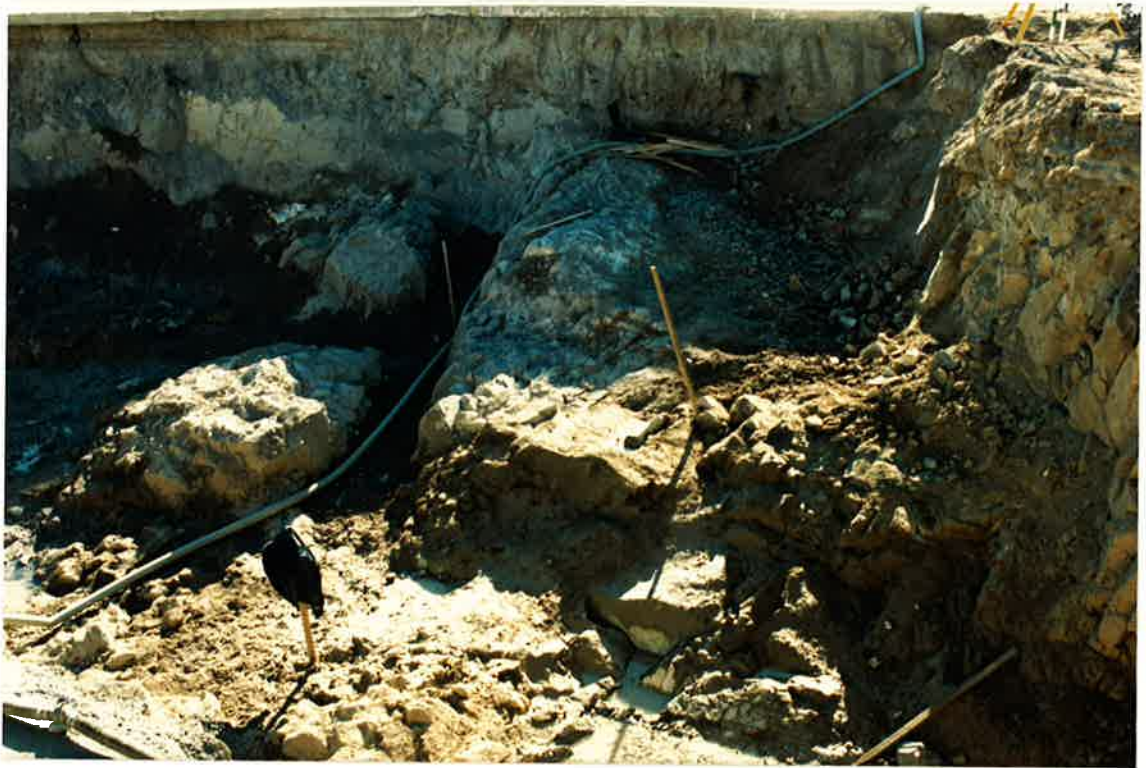
PHOTOGRAPH 4 Southern Abutment, upstream of cut-off trench. June, 1986
