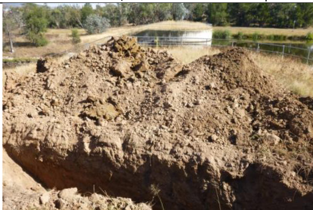
Test Pit T05 – Excavated spoil
