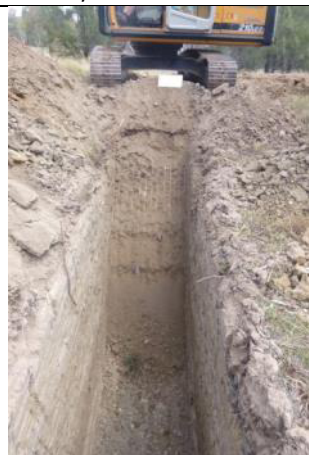
Test Pit T02 – D/S end of Pit
