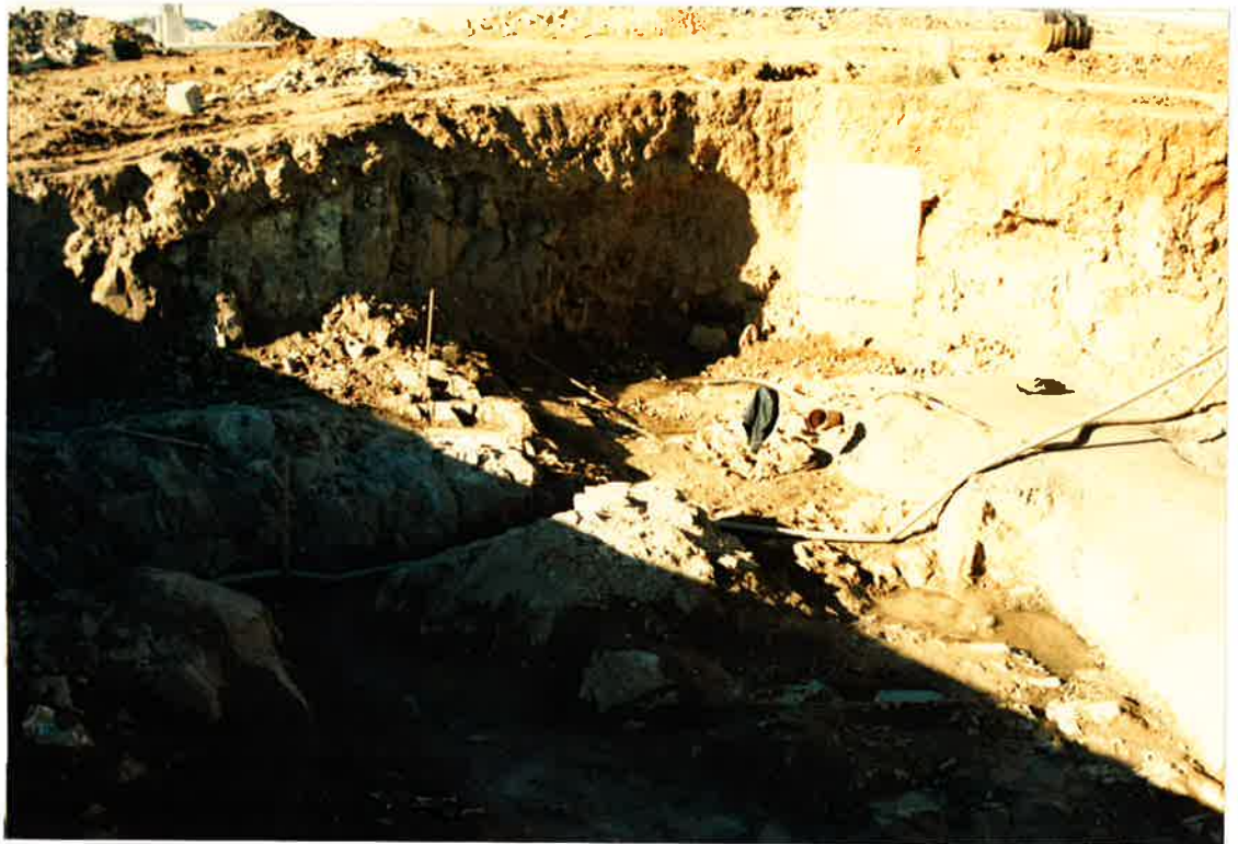
PHOTOGRAPH 5 Southern Abutment, view upstream across cut-off trench. June, 1986
