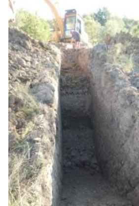
Test Pit T06 – D/S end and right side wall of pit
