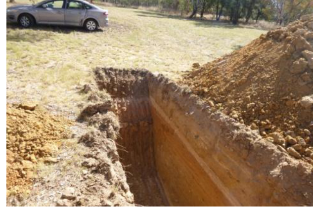
Test Pit T01 – Pit side wall and D/S end
