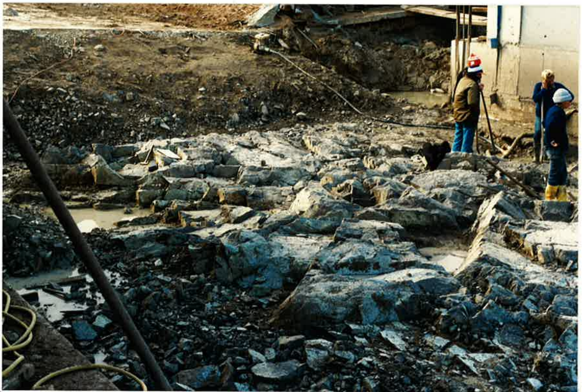
PHOTOGRAPH 13 Central Channel, west side, general foundation clean up. July, 1987
