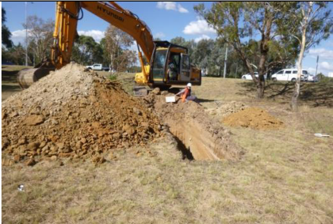
Test Pit T01 – Excavated spoil and general view
