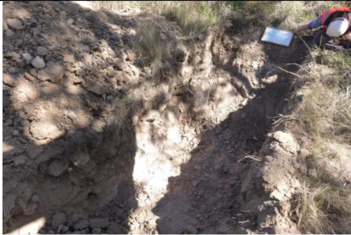
Test Pit T10 –R/H end and D/S side wall of pit (1)
