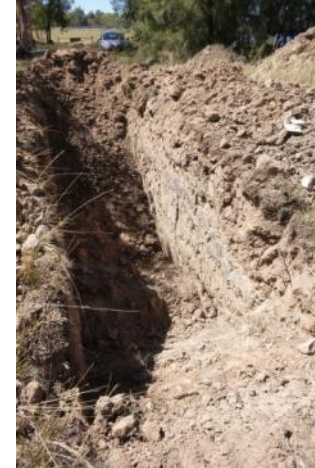
Test Pit T08 – U/S end and left side wall of pit
