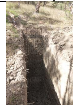
Test Pit T02 –U/S end of pit
