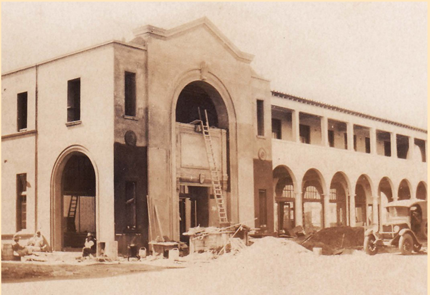
Figure 4 Part of the Sydney Building under construction in 1928. Photo: Archives ACT.
