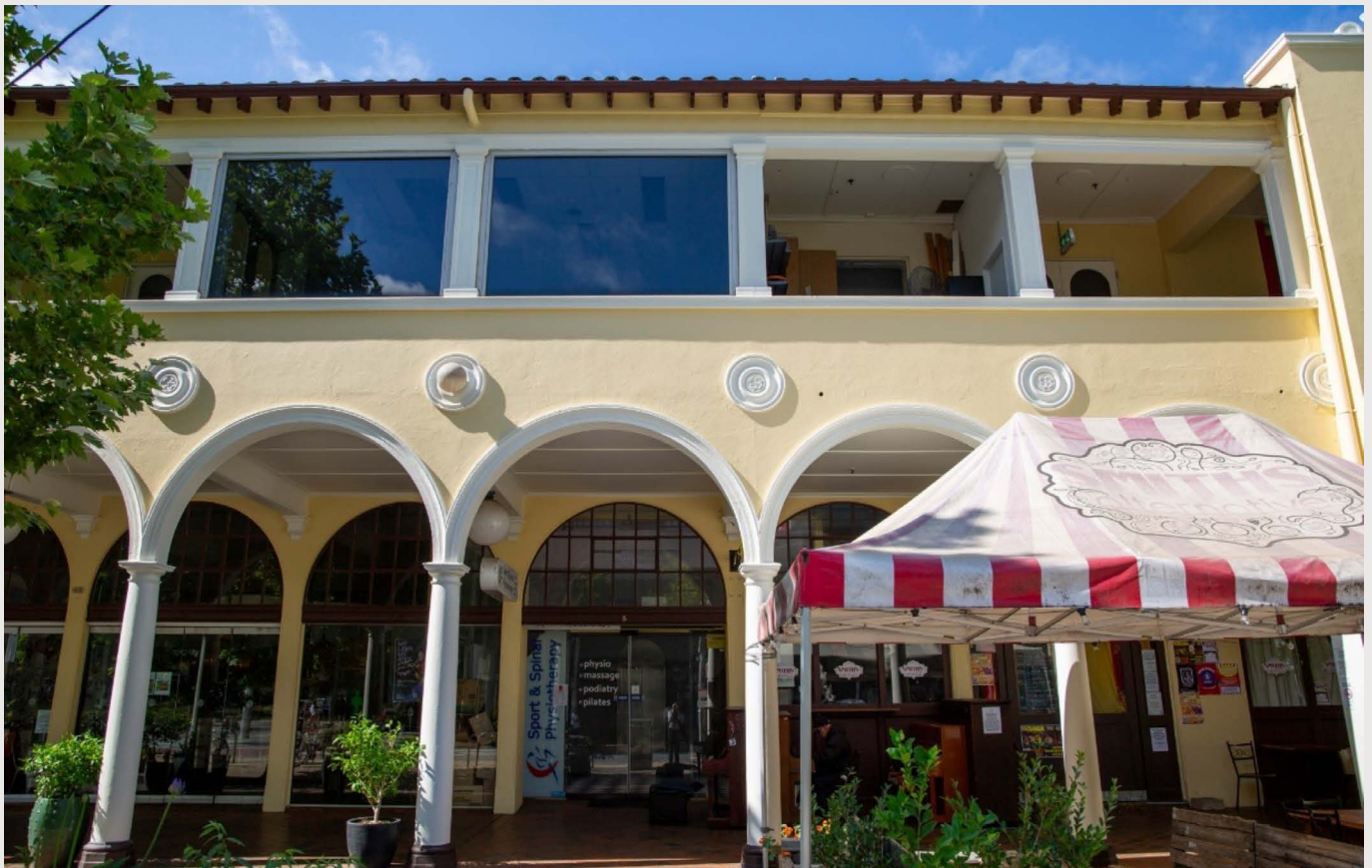
Figure 9 Gutters, downpipes and light fixtures on the Melbourne Building facade at 76-78 Alinga St
