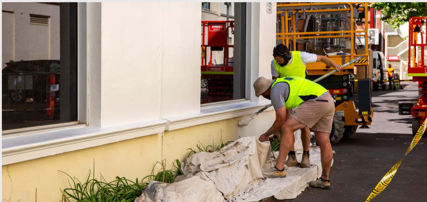
Figure 13 Use of work platforms on public land and temporary traffic management for painting works on Melbourne Building at Odgers Lane entrance
