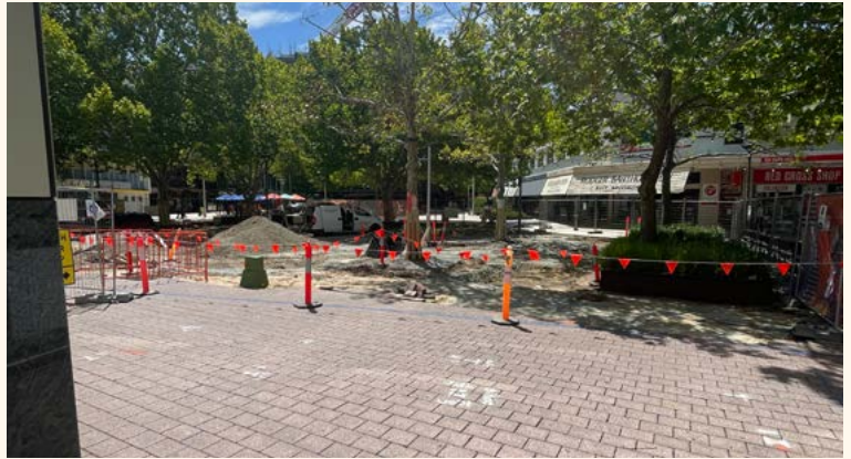
During construction of the City Walk upgrade.
