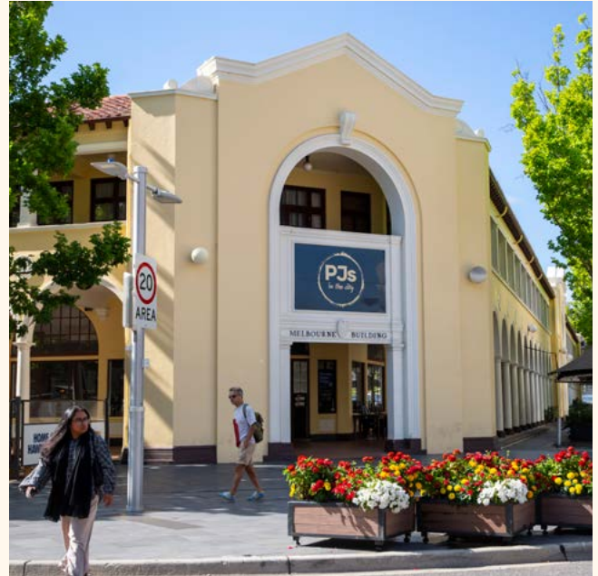
Facades of the Sydney and Melbourne Buildings were repainted in line with the requirements of the Revitalisation Plan.
