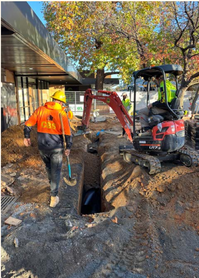
Construction under way on the Dickson Shops upgrade, delivered by Complex Co Pty Ltd from early 2026.
