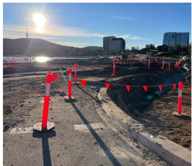
Site works at Acton Waterfront, following lake bed settlement monitoring that confirmed the land is stable for the next stage of construction.
