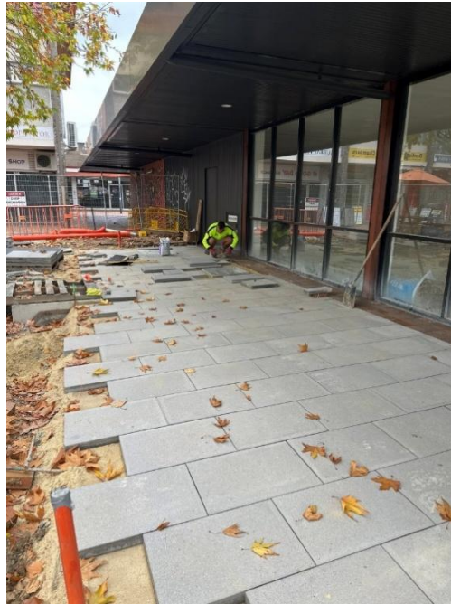
Laying of pavements in Taglietti Square in stage 4a.
