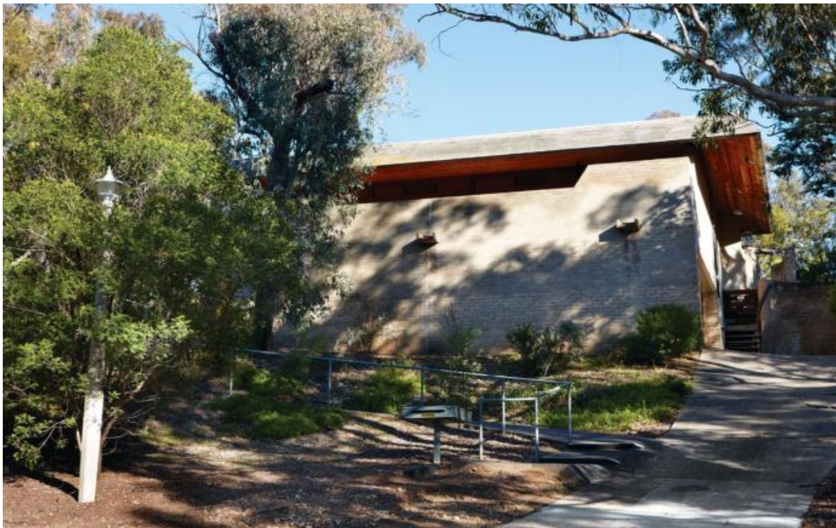
Figure 1: The fortress-like front facade of the house with prominent rainwater spouts (Image: Dianna Snape, see Tanner 2013).
