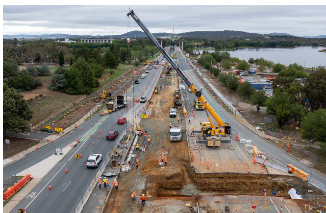
▲ Construction crews installing a new water main beneath Commonwealth Avenue.
