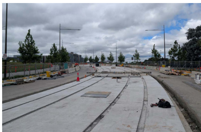
▲ The light rail track slab installed at London Circuit approaching Commonwealth Avenue.
