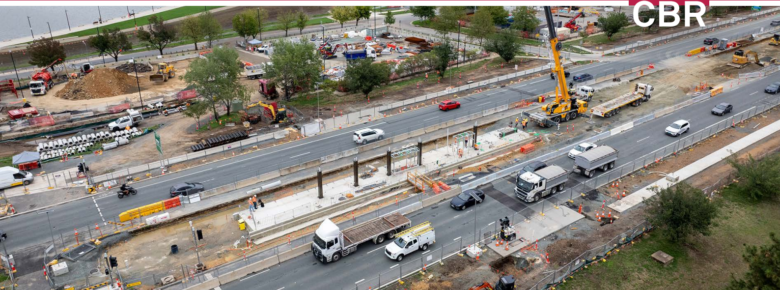
▲ The new Commonwealth Park Light Rail Stop under construction.
