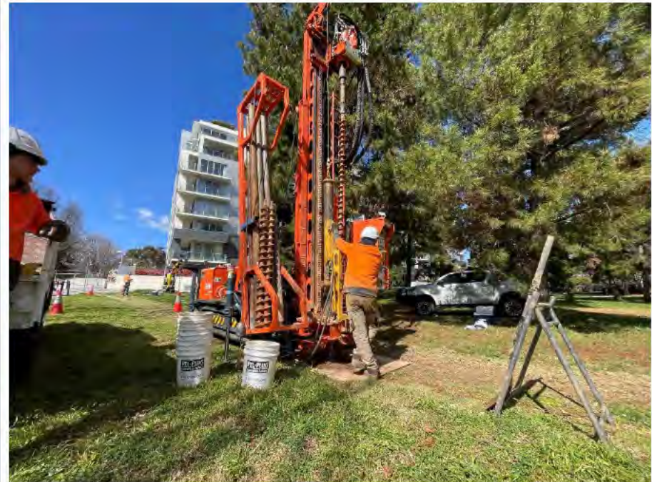
Photo 2 – Drilling at BH24, looking towards south.
