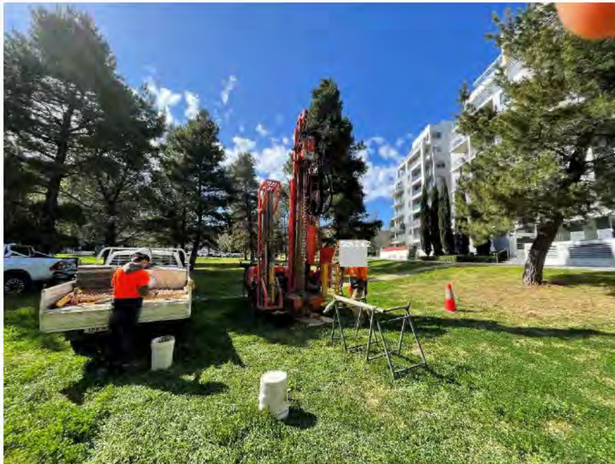
Photo 1 – Drilling at BH23, looking towards north east.
