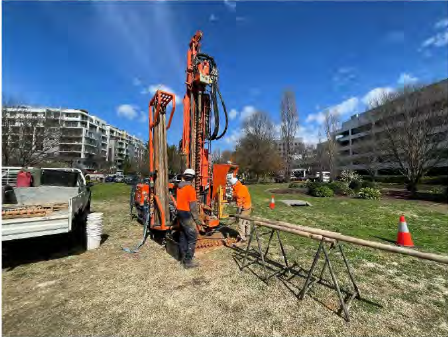
Photo 3 – Drilling at BH25, looking towards south west.
