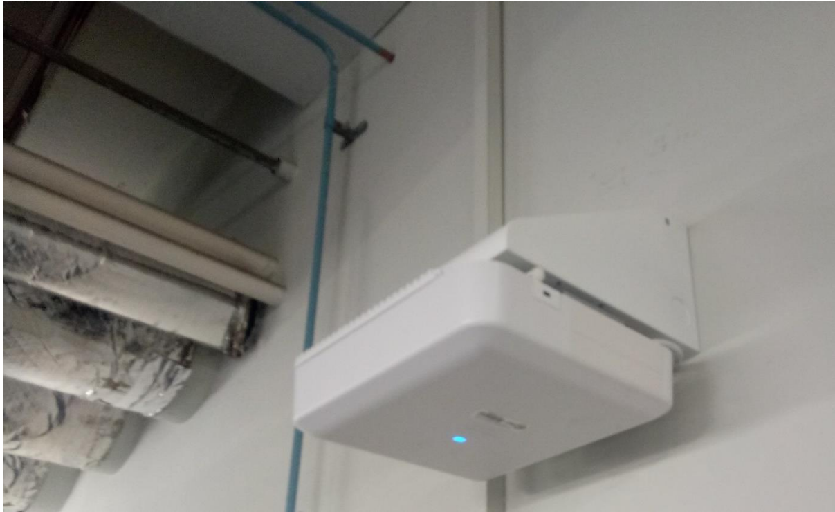
Figure 14 – WAP on a mounting bracket
