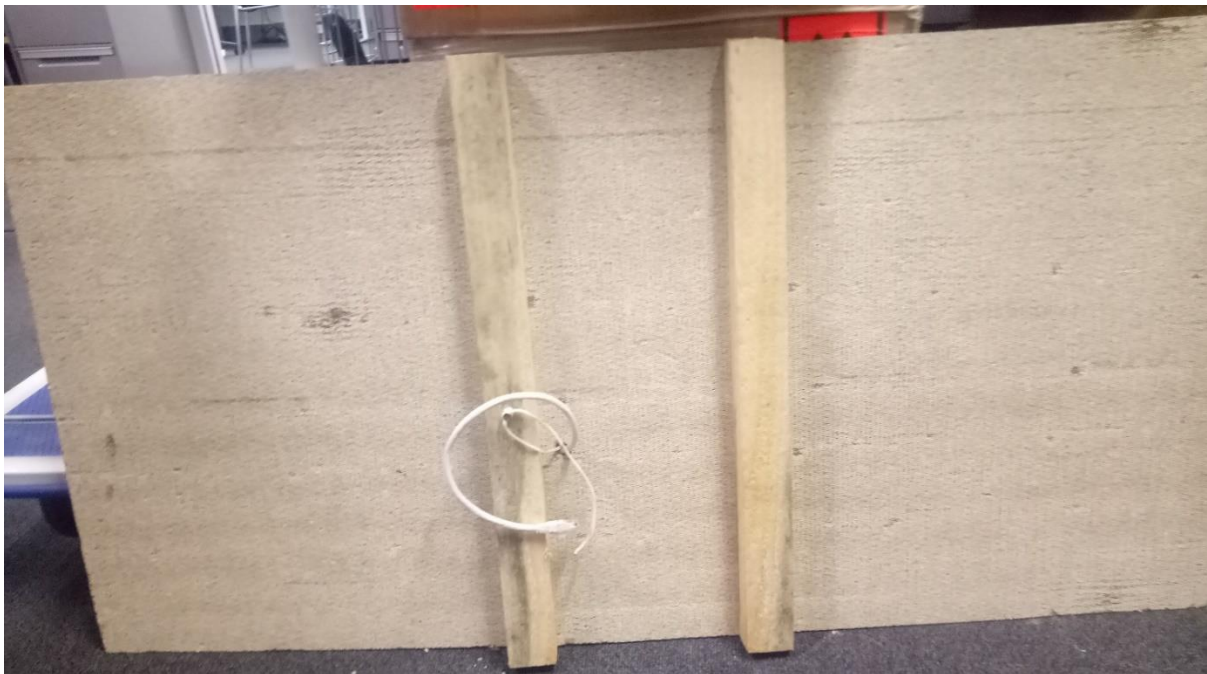
Figure 11 - Wooden Studs for WAP attachment
