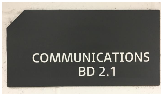
Figure 7 – Building Distributor Communications Room Label – Broad
