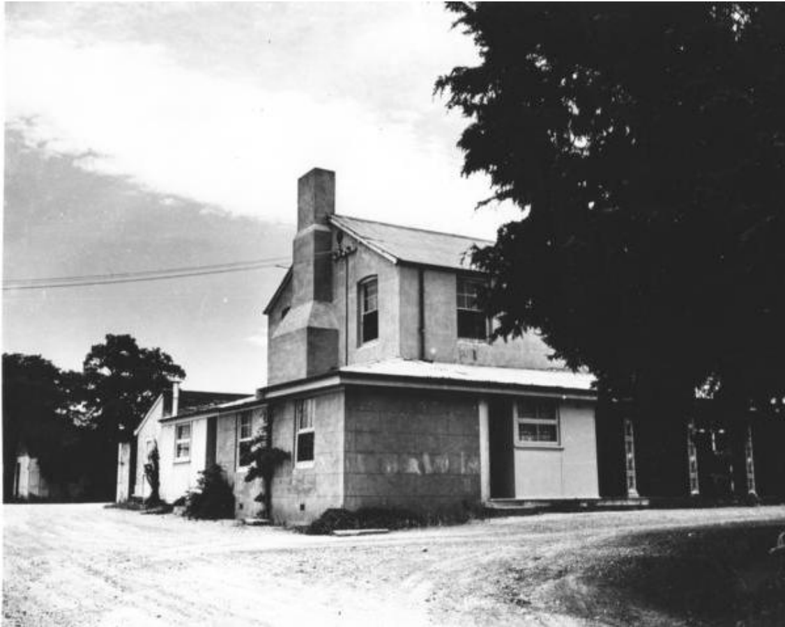
Figure 1: The early section of Gungahlin homestead - built by William Davis (junior), c. 1865, Hall Heritage (n.d.b)
