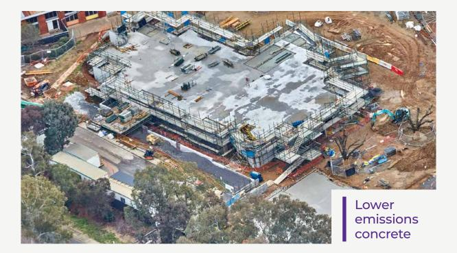
All ground and first floor concrete slabs have recently been completed using the lower emissions concrete, covering approximately 2800m<sup>2</sup> of floor slab.
